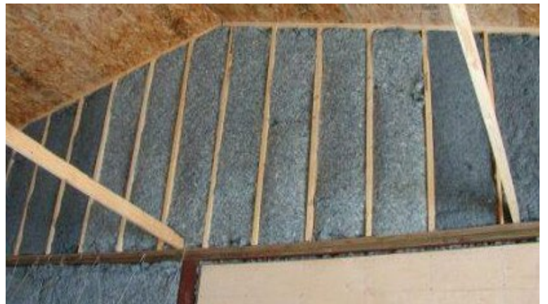
Recycled cotton denim installed as batt insulation in walls.
