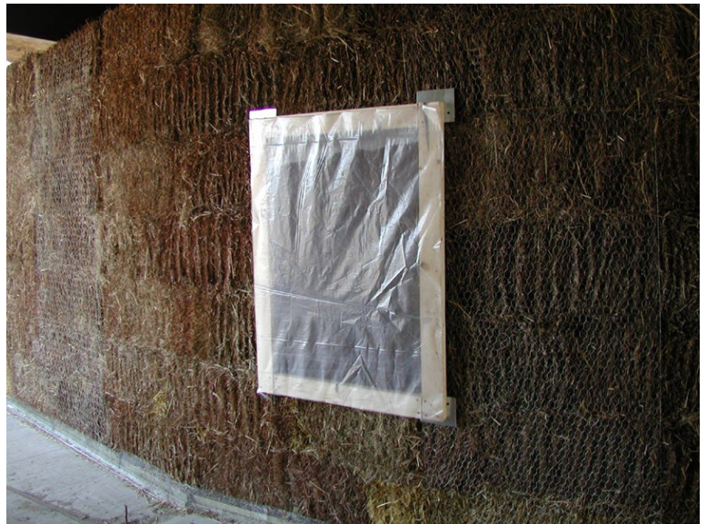
Truth window at north entrance door, surrounded by hay bales.
